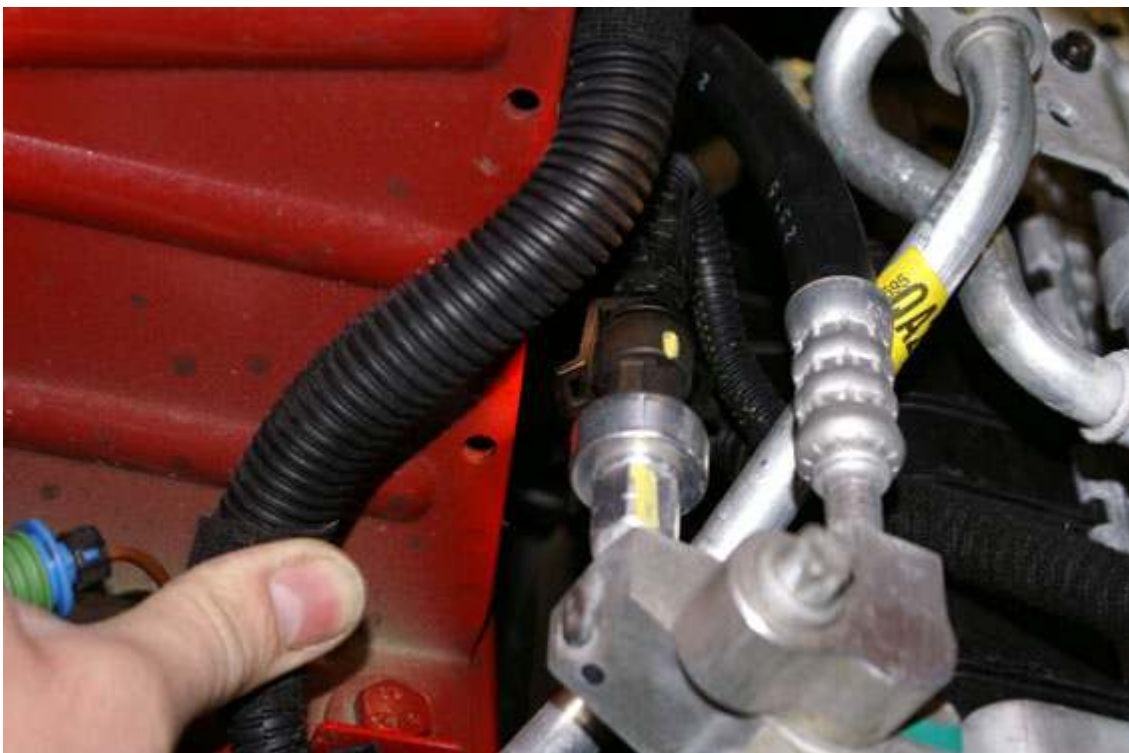
Picture 6 - Aircon Valve Clearance - Check.
